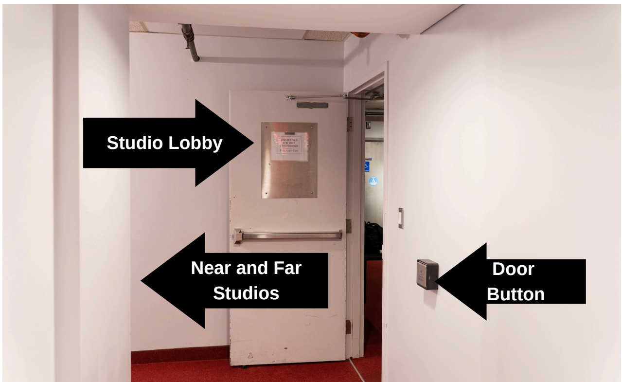
[image of the Studio Lobby door with arrows pointing towards the "Studio Lobby" and "Far Studio"]
